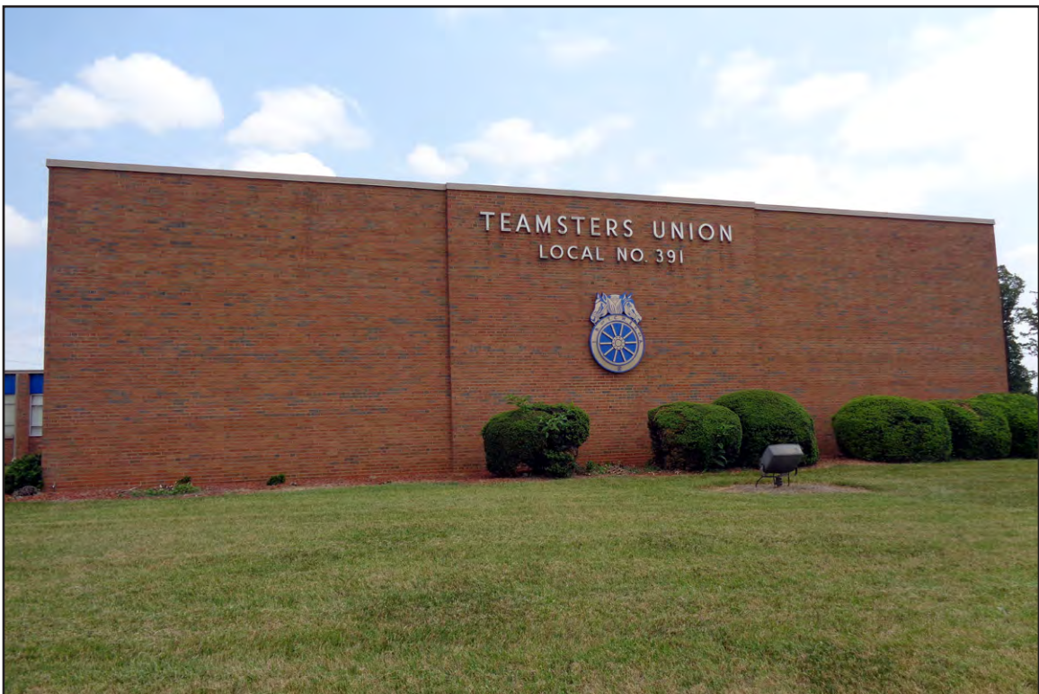
PLATE 4: Chauffeurs and Teamsters Union Local 391 Building, Eastern End, Looking North
