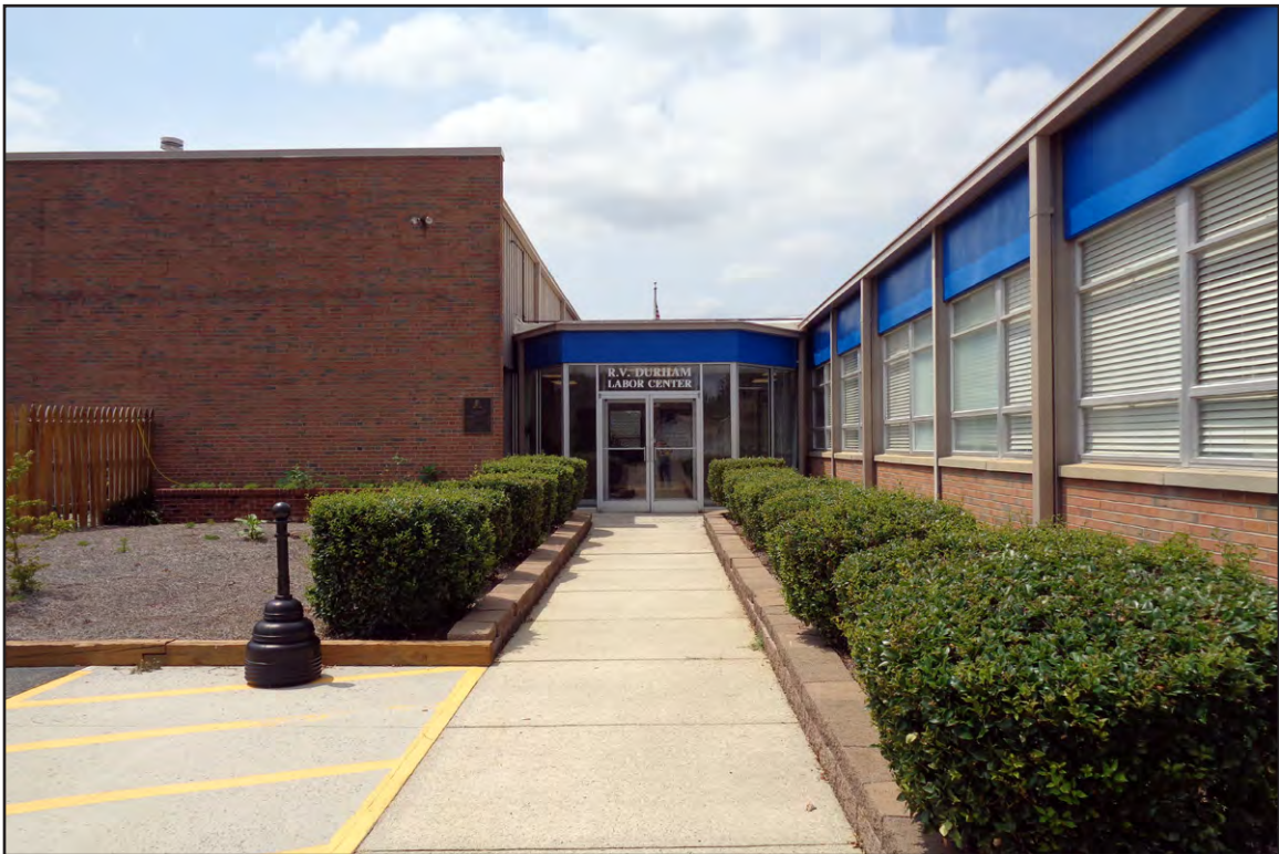
PLATE 8: Chauffeurs and Teamsters Union Local 391 Building, Front Entrance, Looking Southwest
