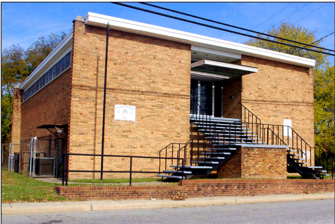
PLATE 20: Toussaint L'Ouverture Lodge No. 524 (GF7022), High Point, Looking North
