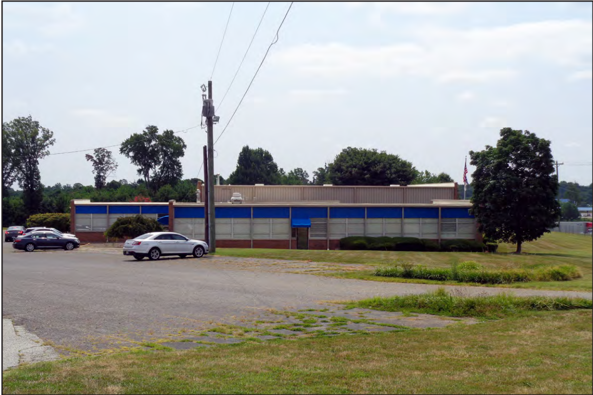
PLATE 1: Chauffeurs and Teamsters Union Local 391 Building, Looking East
