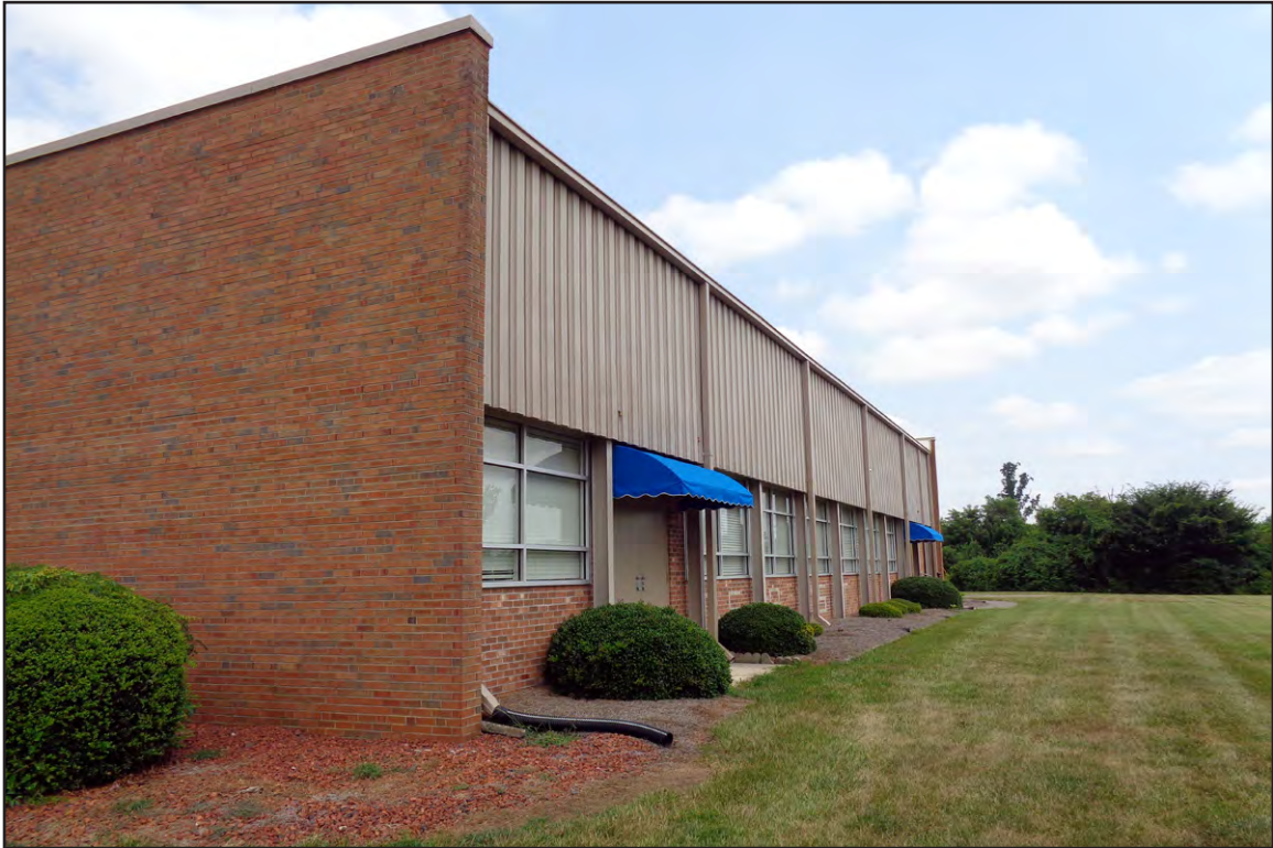
PLATE 5: Chauffeurs and Teamsters Union Local 391 Building, Looking Northwest
