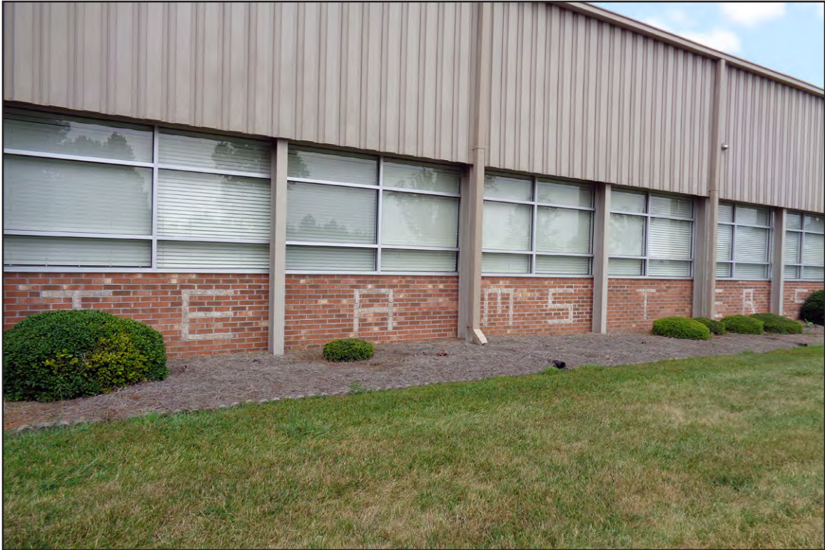
PLATE 7: Detail of Decorative "Teamsters" Brick Work on East Elevation
