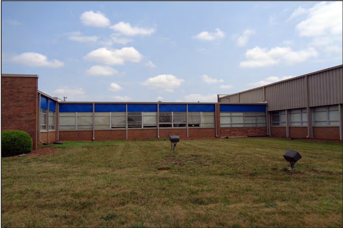
PLATE 3: Chauffeurs and Teamsters Union Local 391 Building, Central Section, Looking North
