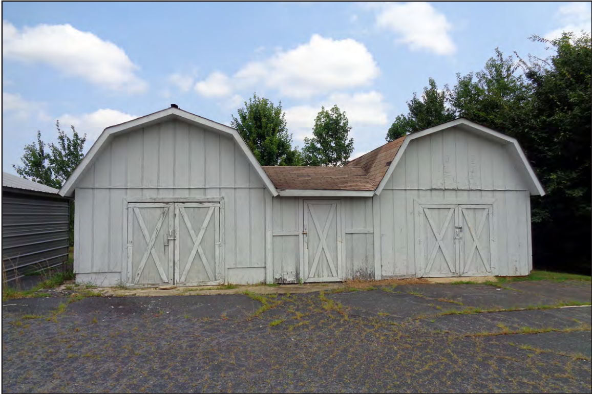
PLATE 13: Shed Outbuilding, Looking North
