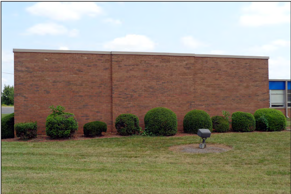
PLATE 2: Chauffeurs and Teamsters Union Local 391 Building, Western End, Looking North
